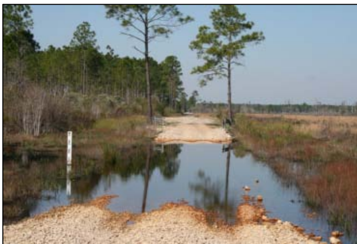
Figure 2. Low water crossing
