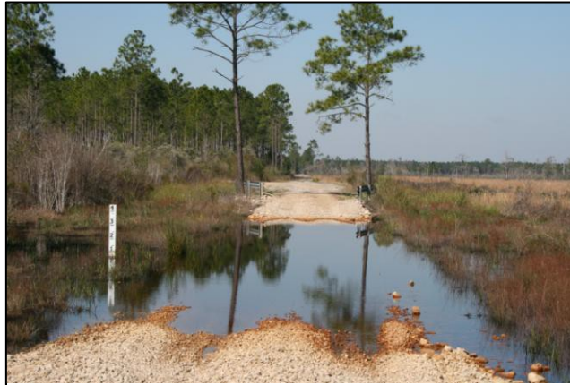
Figure 3. Low Water Crossing
